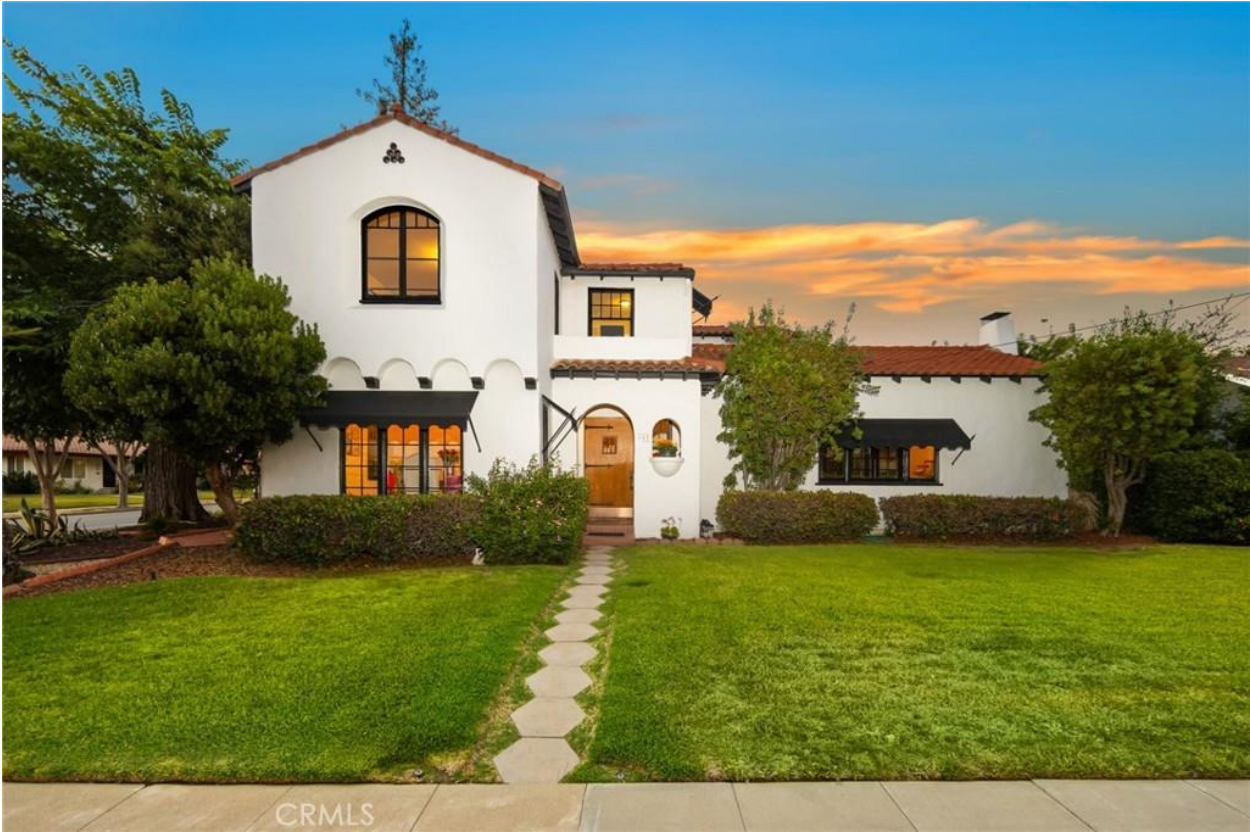
Front of Home (South Elevation)
