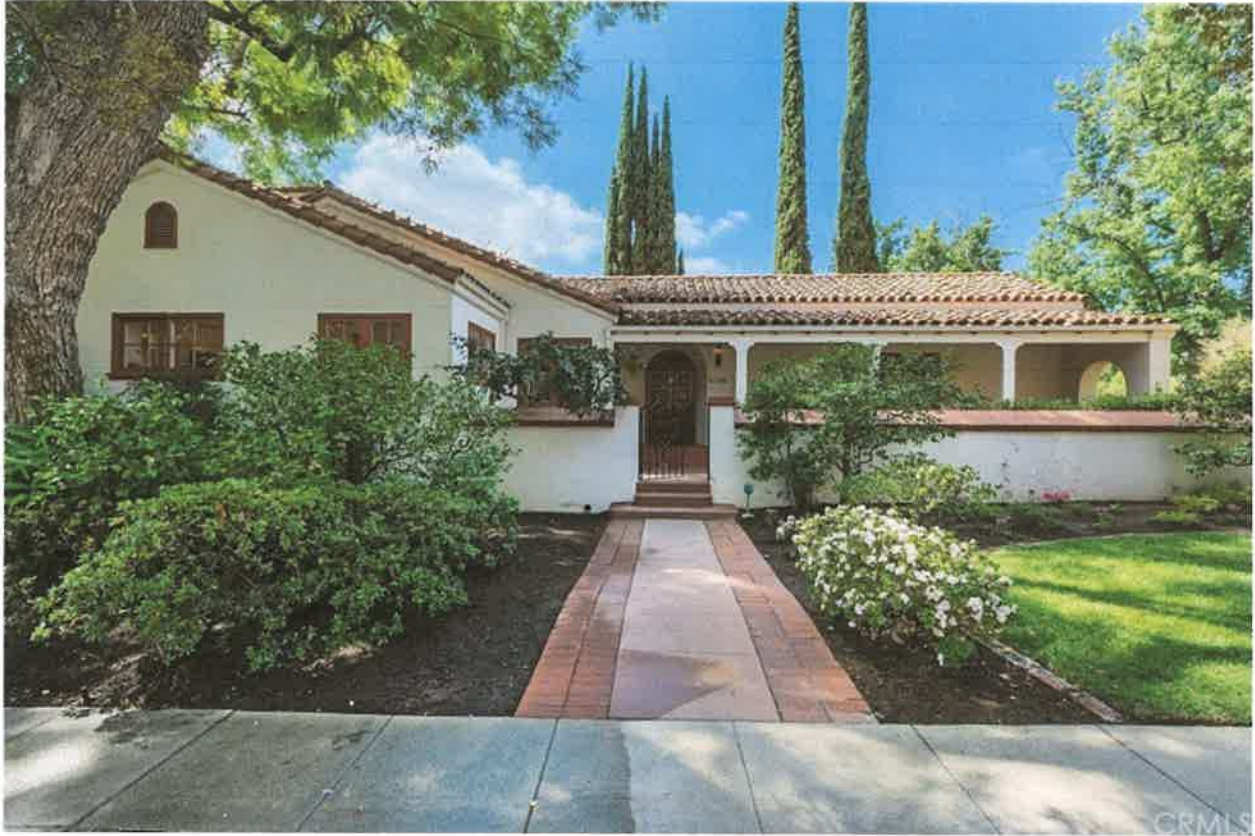
View of the East side of the property (Circa, 2019)
