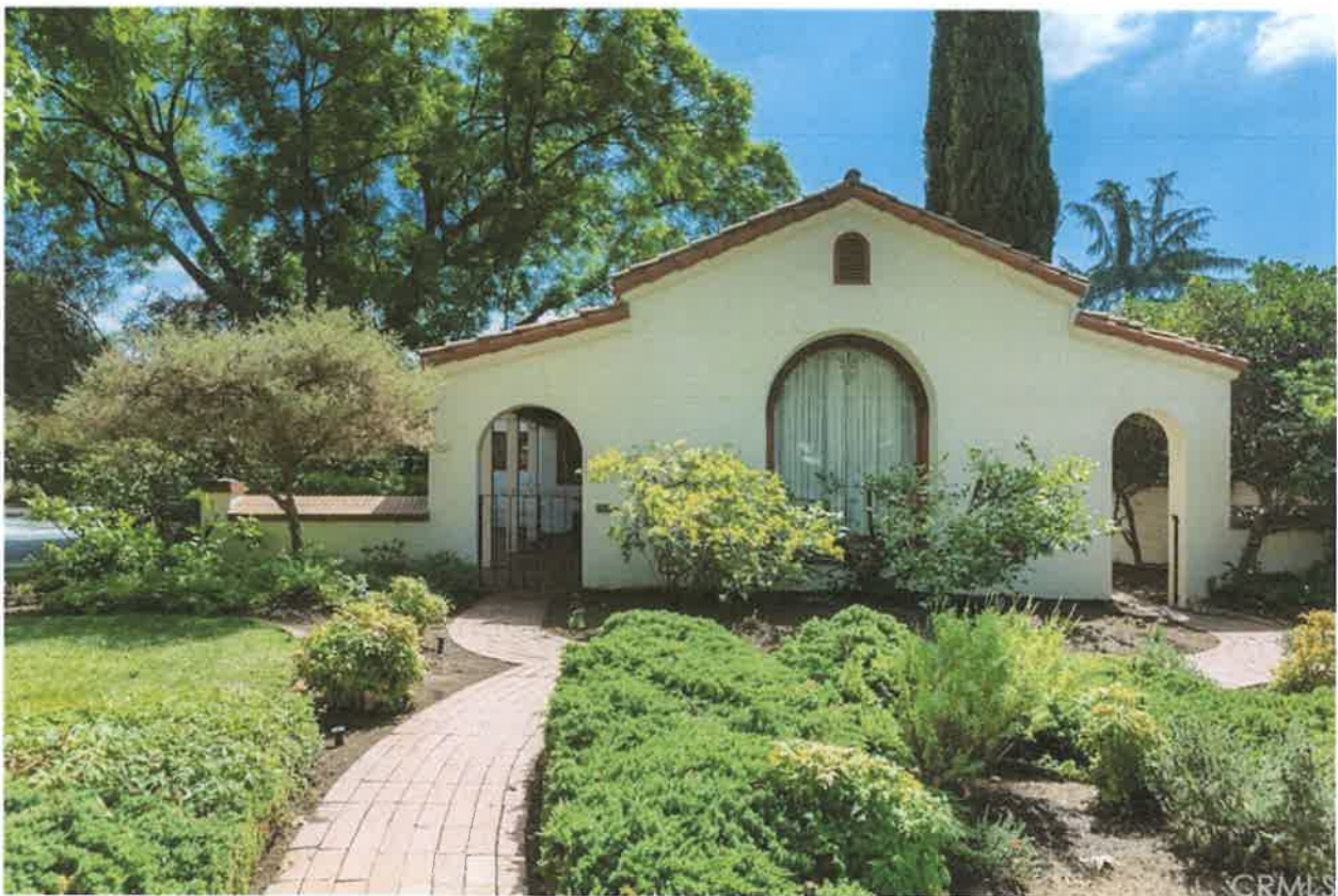
View of the North side of the property (Circa, 2019)
