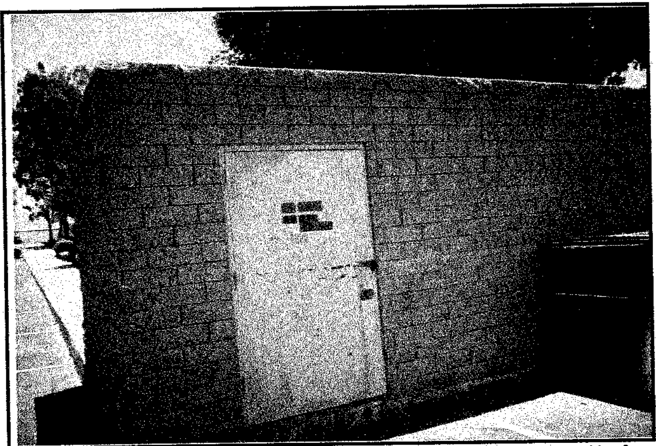
Photograph #3 East facing view of the electrical service and transformer building. Inside of this room are four transformers, which are owned by Southern California Edison.
