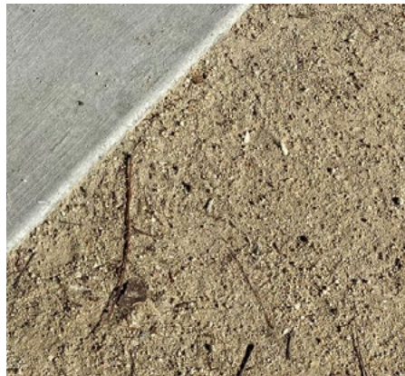
Decomposed Granite Loose
