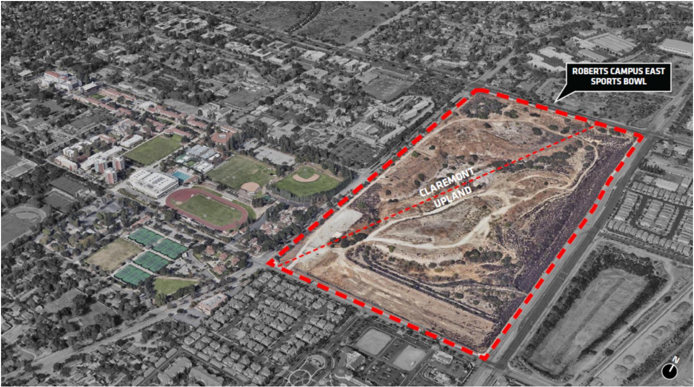
Aerial View of East Campus Site
