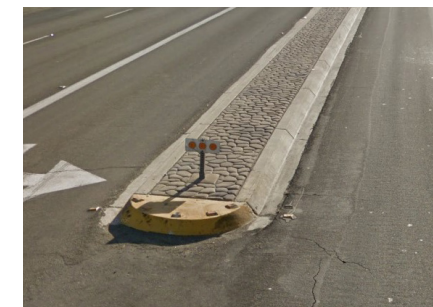
Concrete separator for access management (2')
