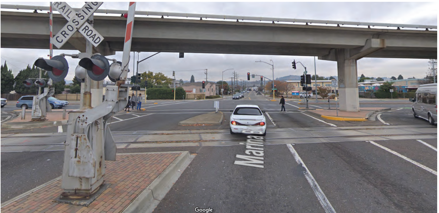
The BART aerial crossing at Marina Boulevard in San Leandro, CA mimics the proposed Garey Avenue crosswalk, with at-grade freight rail, aerial light rail and a crosswalk in close proximity.
