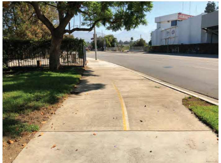
The existing side path on Fairplex Drive is not used by most cyclists.
