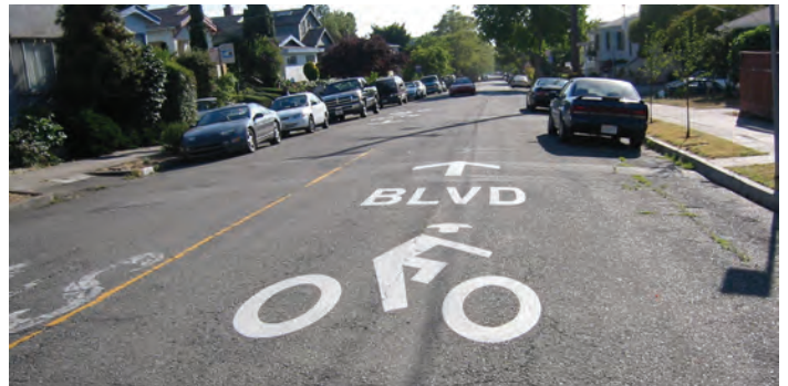
Bike boulevards allow motorists traveling at slow speeds and cyclists to share the roadway.
