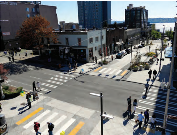
Shared streets use paving, planted medians and subtle turns in the vehicular path to slow vehicles to the point that they can safely share space with pedestrians and cyclists.
