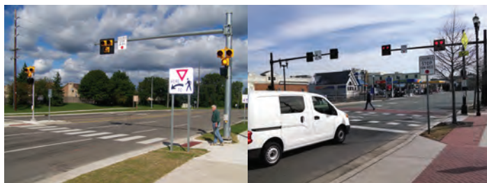
Crossings of major streets should be highly visible and safe. A HAWK signal is suggested for the intersection of 5th Street and San Dimas Avenue.
