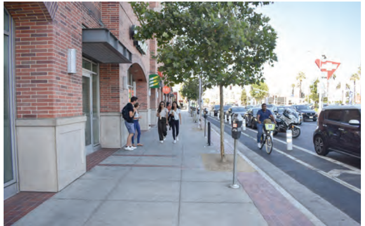
Landscaped curb extensions would be helpful on the north leg of the Glendora Avenue and Route 66 intersection. They would protect pedestrians and cyclists at intersections and serve as a gateway treatment. Beyond the gateway, bike lanes can be protected by lower-cost solutions such as bollards.
