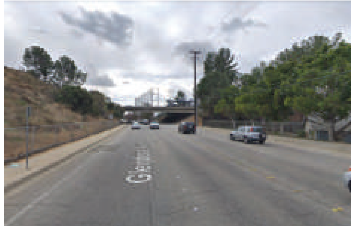
View of Glendora Avenue at the 210 Freeway overpass.
