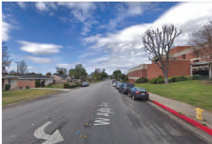
Portions of Ada Avenue near Foothill Presbyterian Hospital have no sidewalks.
