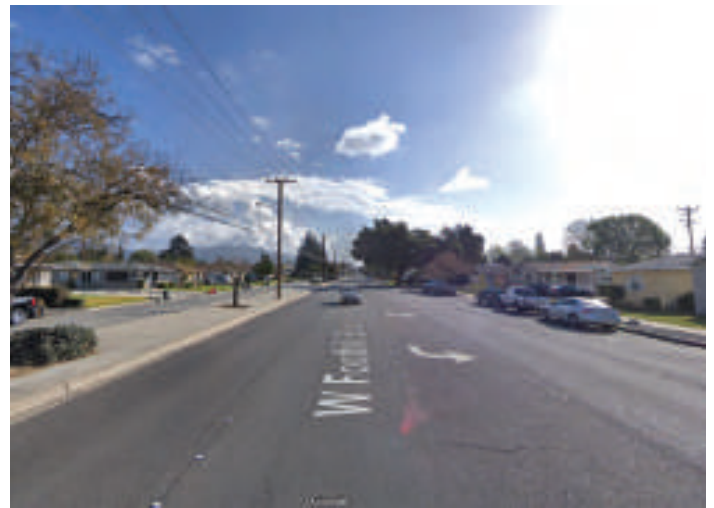
A portion of Foothill Boulevard west of Grand Avenue already has only one eastbound lane, due to a narrower right-of-way.
