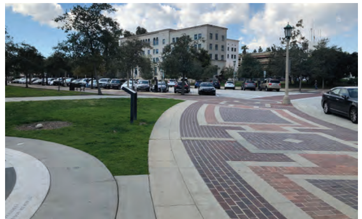
A special paving pattern can be used to guide pedestrians along the pathway.
