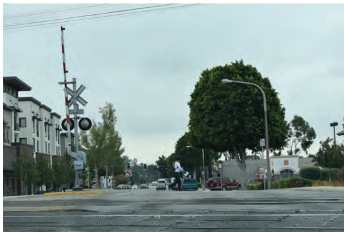
Reducing traffic lanes will increase the safety of the new crosswalk to be located at the Gold Line tracks.
