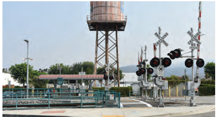
View of the future Pomona North station site
