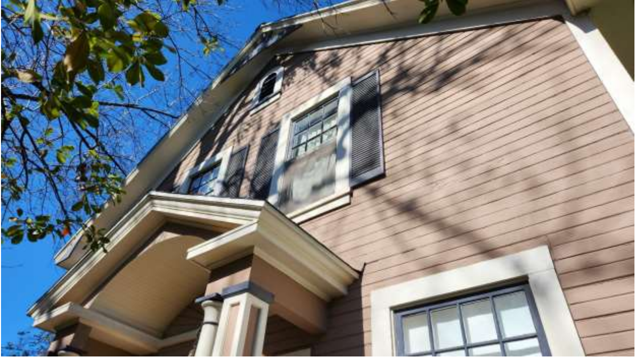
Wood Frame Divided Windows and Louvered Shutters
