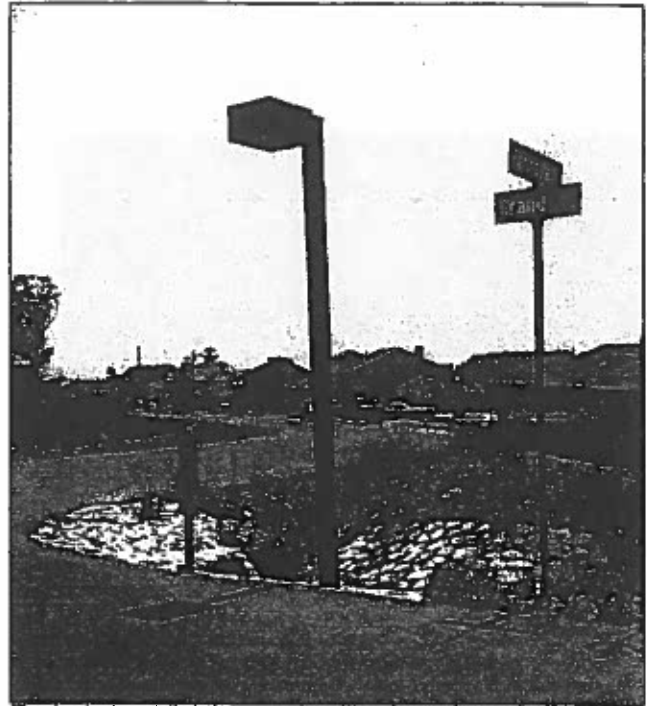
Typical street lighting used to illuminate intersections and stop signs only.
