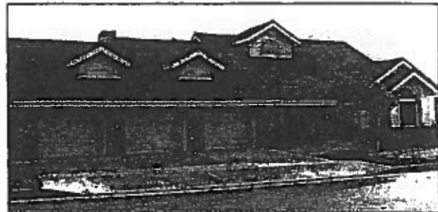
Inappropriate. The artificial dormers on the garage have no function.
