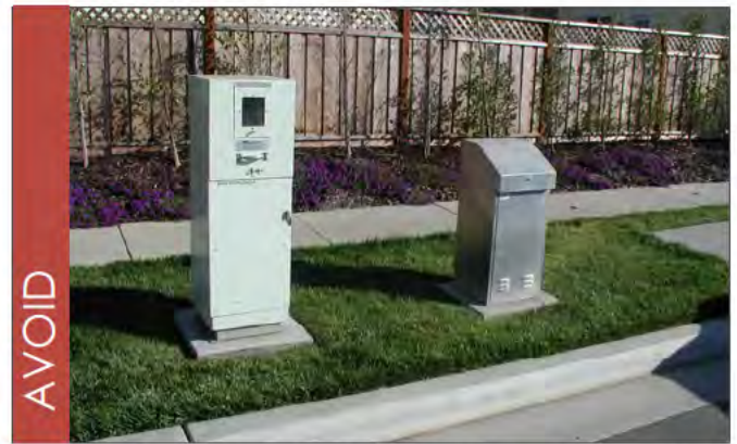
Example of inappropriately placed utility boxes in a parkway.
