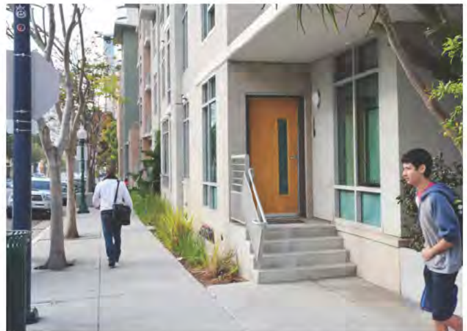
Recessed stoop with primary entry perpendicular to the street for added privacy.
