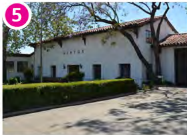
The Vortex building preserves a piece of Village South's history, and will be adaptively re-used as a new community-gathering place.
