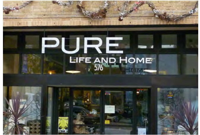
Wall signs may be located within the transom area of the shopfront.
