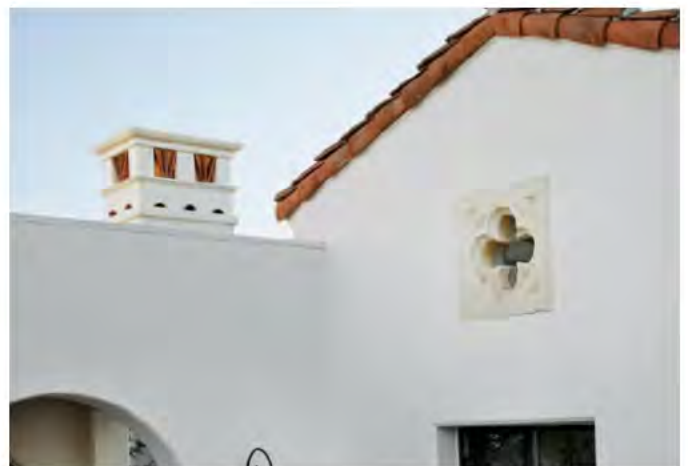
Gabled roof with decorative tile on the gable façade
