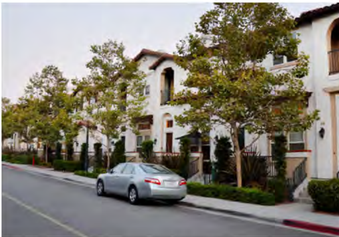
A stucco building with tile roof - a flat roof is screened by Parapet walls faced with a pitched roof.
