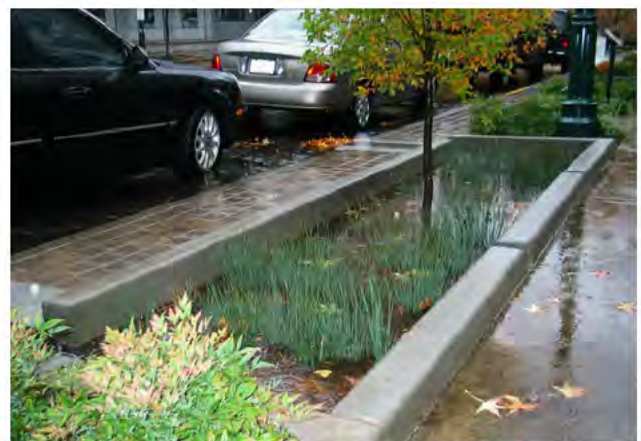
Village South's public realm network is an integral part of its stormwater management plan.
