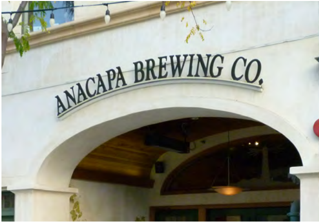
Individual metal letters mounted on a string course.
