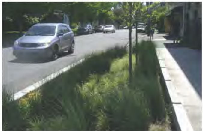
Rain gardens with curb cuts help manage runoff from rain events.
