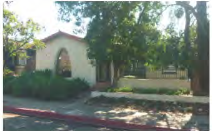
194 S. Indian Hill Blvd. is a single-family residence that was constructed in 1930. Its historical integrity is well-preserved, with very little modification.
