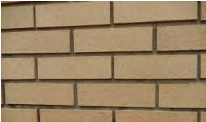
Mortar joints are raked.
