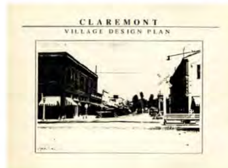
Claremont Village Design Plan (1987): documented the character-defining urban patterns of the village and provided design guidelines to ensure future additions and improvements "enrich and preserve the Village."
