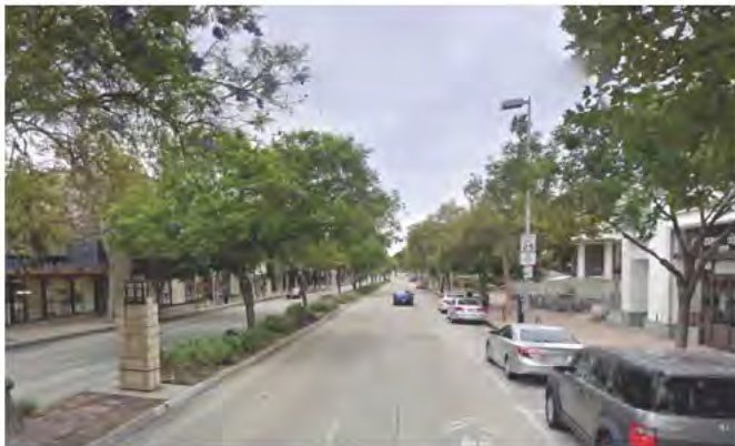
Two travel lanes in each direction with a center median, on-street parking, and possible sharrowed outer lanes.
