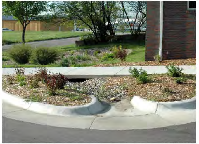
A bulb-out containing a swale with access to street runoff
