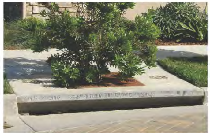
Storm drain filter systems help to naturally filter runoff.
