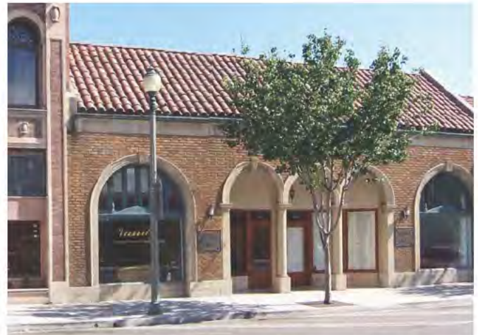
A masonry shopfront with an arcaded entrance and display windows
