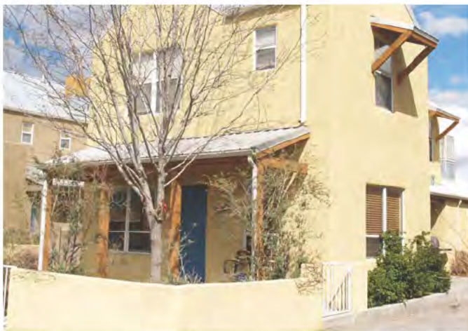
Brackets support a metal window awning.
