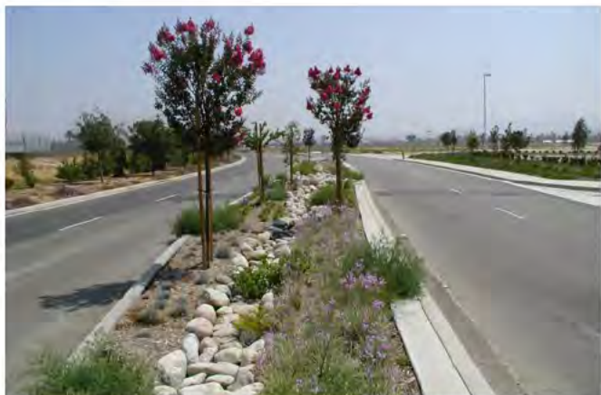
A median with a small river stone drainage bed and drought-tolerant plants
