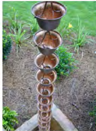
Rain chains help to divert and store rainwater from gutters
