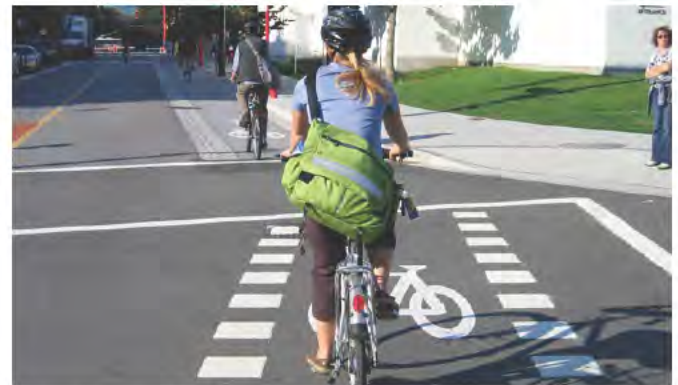
Clearly marked bike Crossings at intersections for improved safety.
