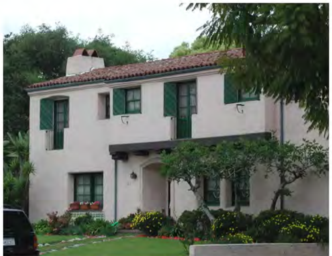
A Spanish Revival courtyard building with a portion of the second floor cantilevering over the front entry
