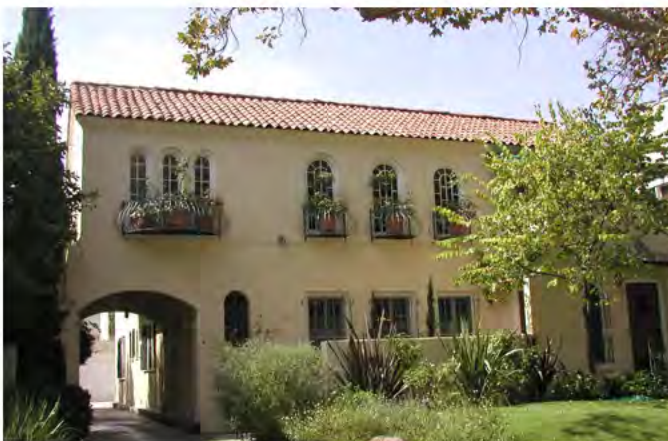
A Spanish revival porte cochere that is designed to be an integral part of the building
