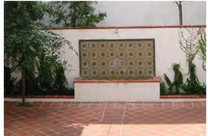
Smooth plaster walls may incorporate decorative tile or terra cotta accents. These walls also have a cap.
