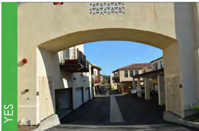
Example of mechanical equipment well-screened by an architectural element incorporated into the building's composition.
