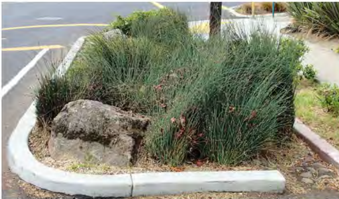
Corner bulb-out planter with street drainage maintained
