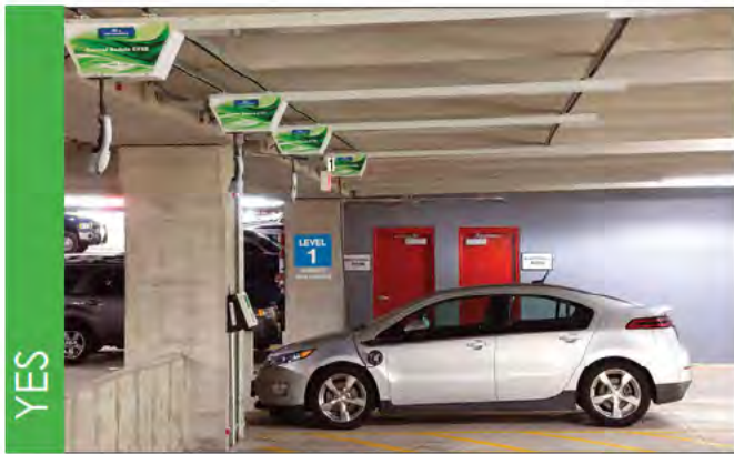
Wherever possible, mechanical/utlities equipment should be placed in mechanical room, typically accessible from the building's parking lot/structure.
