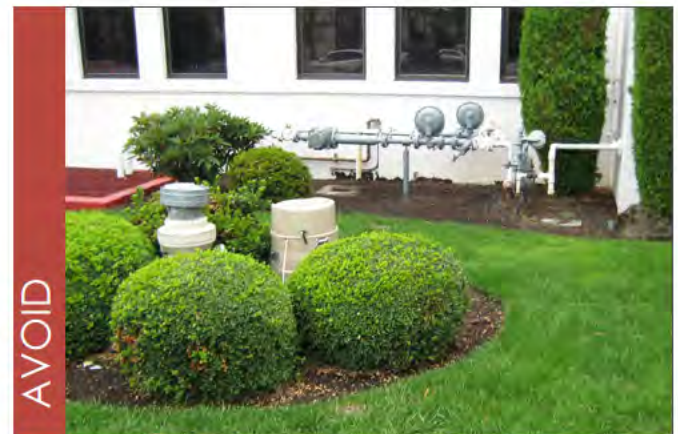
Example of inappropriately placed check valves and other utility devices in the front yard of a commercial building and in a parkway.
