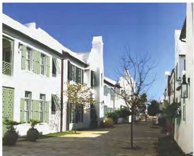
A paseo with flagstone and embedded planters that receive runoff
