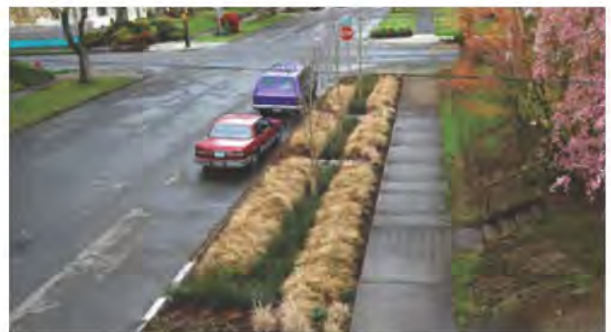
Parkway Bioswales: Create a "buffer" between pedestrians and moving traffic and provide stormwater retention & infiltration.
