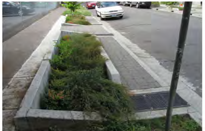
Drainage channels may be cut into street curbface to allow street run-off water to drain into bioswales, providing biofiltration and wastewater management.
