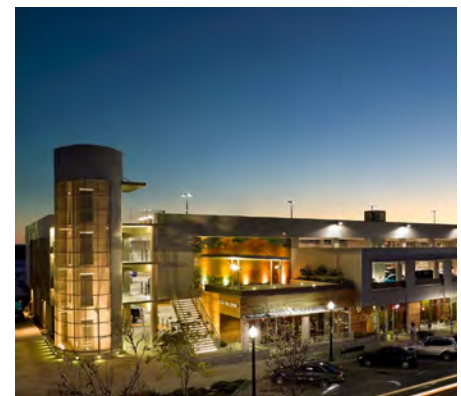
1st Street Garage: The structure on First St is a fine example of an actively lined shared parking structure.
