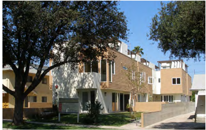
Multiple roof decks on one building.
