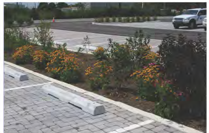
Parking with permeable pavers and rainwater collecting planters
