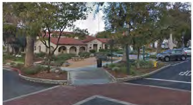
Corner & Mid-Block "Bulb-outs": Enhance pedestrian safety and provide street landscape and stormwater retention & infiltration.
