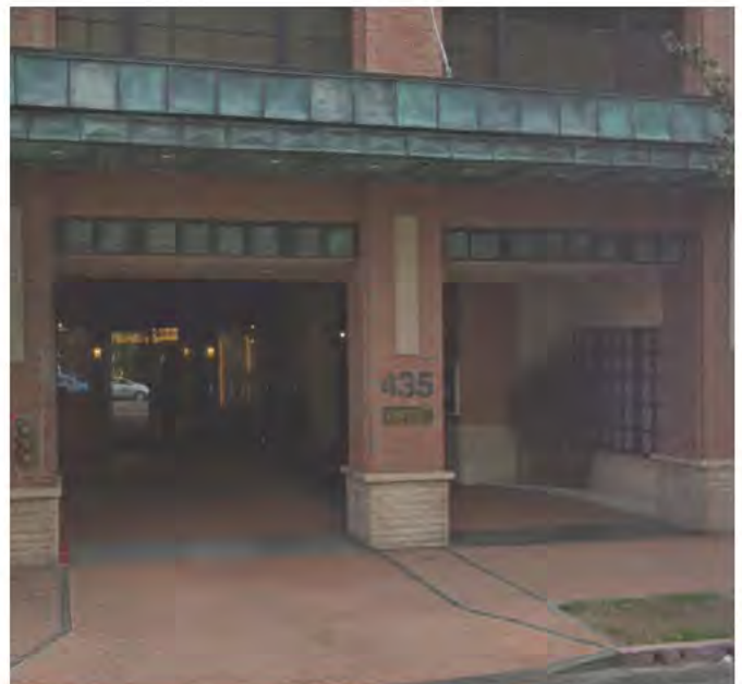
The vehicular entrance to this structure is as narrow as practicable, and separate from the pedestrian entrance. The attention to aesthetic detail matches that of the rest of the building.
