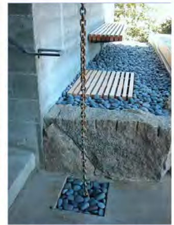
Rain chains help to divert and store rainwater from gutters
