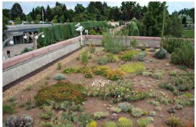
Green roofs are used to capture and store water on-site.
