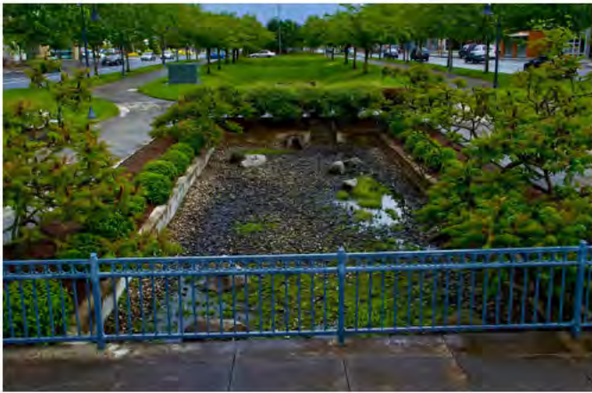
Stormwater area appropriately integrated within a park.
