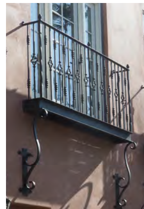
Projecting Metal Balconies
