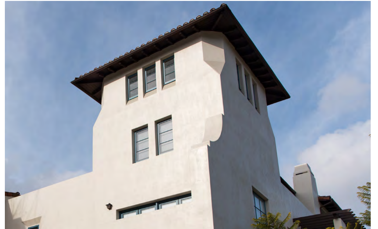
Tower as architectural accent.
