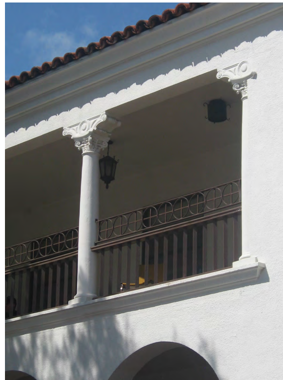
A loggia brings natural light into an upper story circulation path and views into courtyard.
