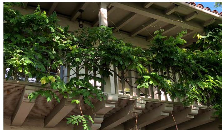
Wood Balconies, Posts, and Rafters
