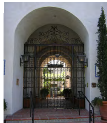
Paseo and Metal Gate
