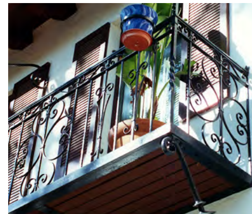
Projecting Metal Balconies
