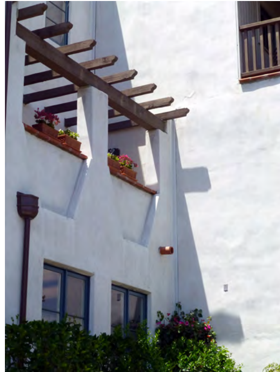
Trellis shades residential terrace while enhancing the visual interest of the building elevation.
