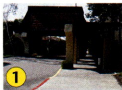
1 Existing Hotel Lobby Entrance
