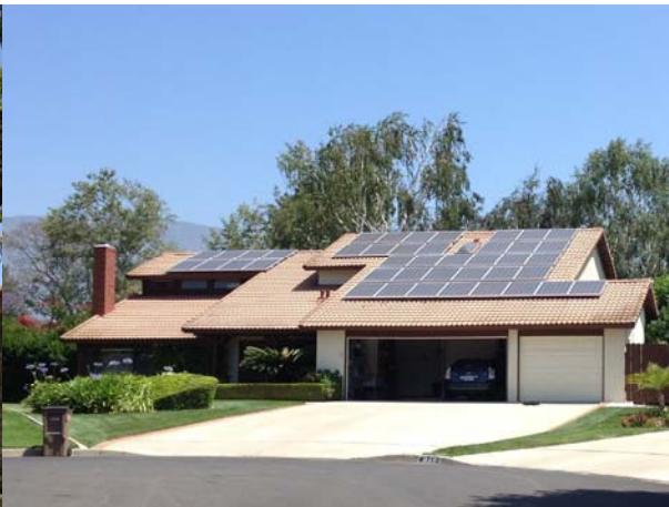
Home Solar System
