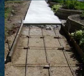
Reinforced or Thicker Slab
