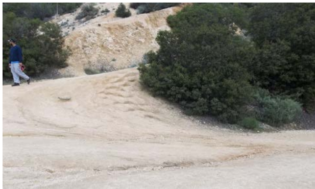
Evidence of switchback cutting Source: City of Claremont
